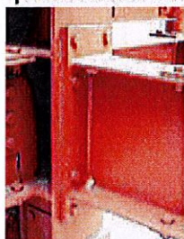
Extended end-plate connection
